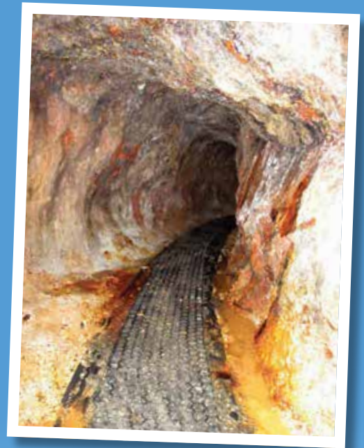
A flash photo inside a portion of Collins Drive tunnel shows a bend that obscures the tunnel's exit portal. Gone are the slippery wooden planks on the floor, replaced with more stable rubber mats.
