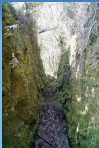
Parts of the water race are actually hewn from solid rock.
